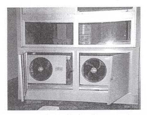
The above picture is of the two Fujitsu air conditioner compressor/condenser units installed in a sound insulated cabinet within each demountable class room. There is only external access to the units.
